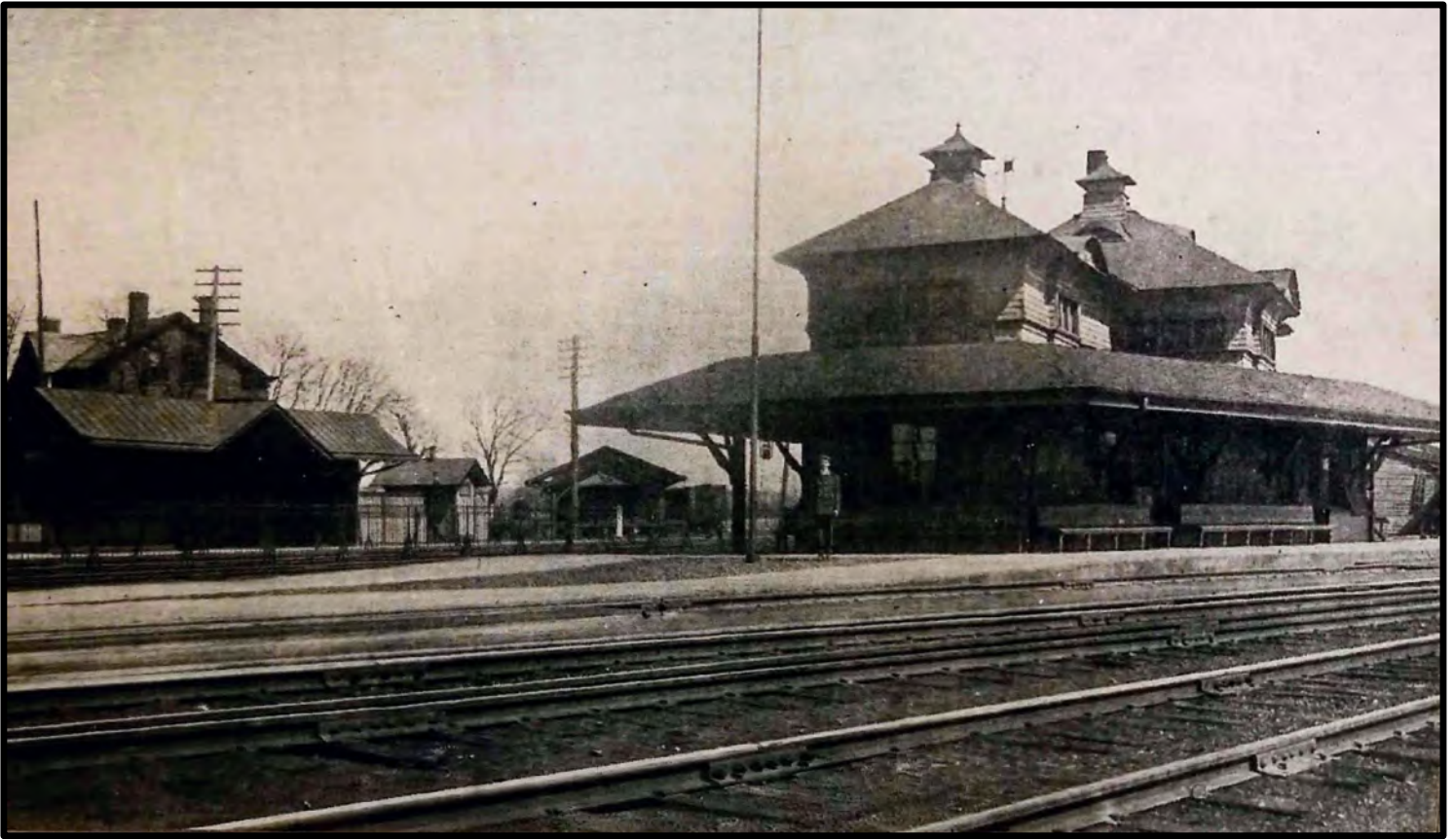
Figure 5: Historical Monmouth Junction Station Photo 2
