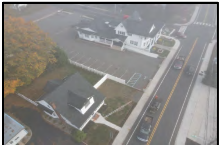
620-616 Ridge Road (House + Funeral Home)
