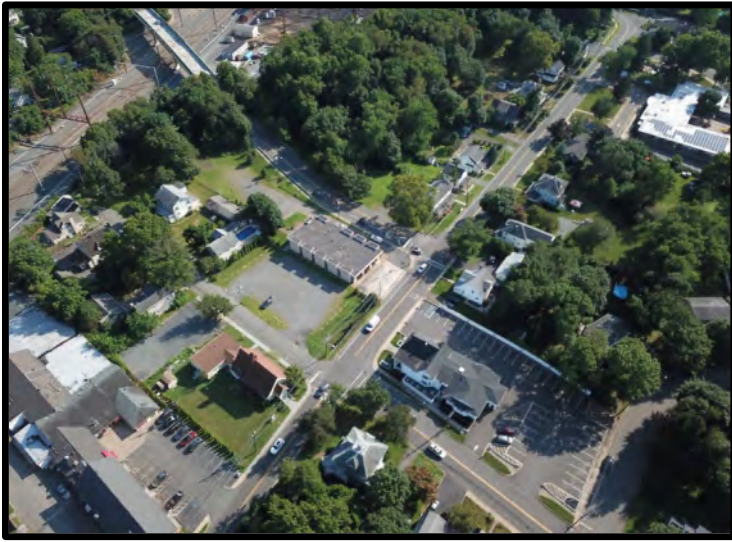
Ridge Road / New Road Intersection
