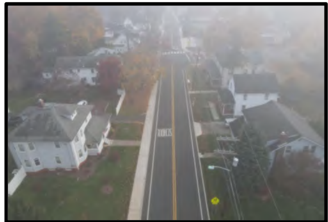
624 + 629 Ridge Road (Viewing East)
